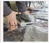
**3.** Staple the insulation at minimum 300mm intervals, maintaining a 50mm overlap between layers.
