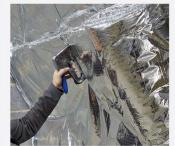
**4.** Tape and seal the perimeter and overlaps using *ThermaSeal* Foil Tape, creating an airtight vapour control barrier.
