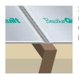
**1.2** Begin the next roll from this rafter, by butt-jointing it to the end of the first roll and staple in place.
